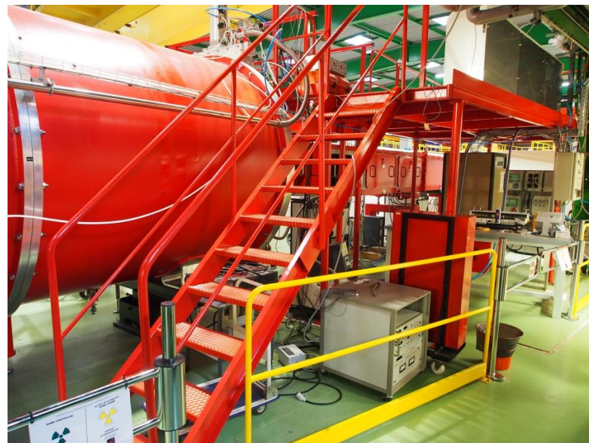
Platform for top access & storage
